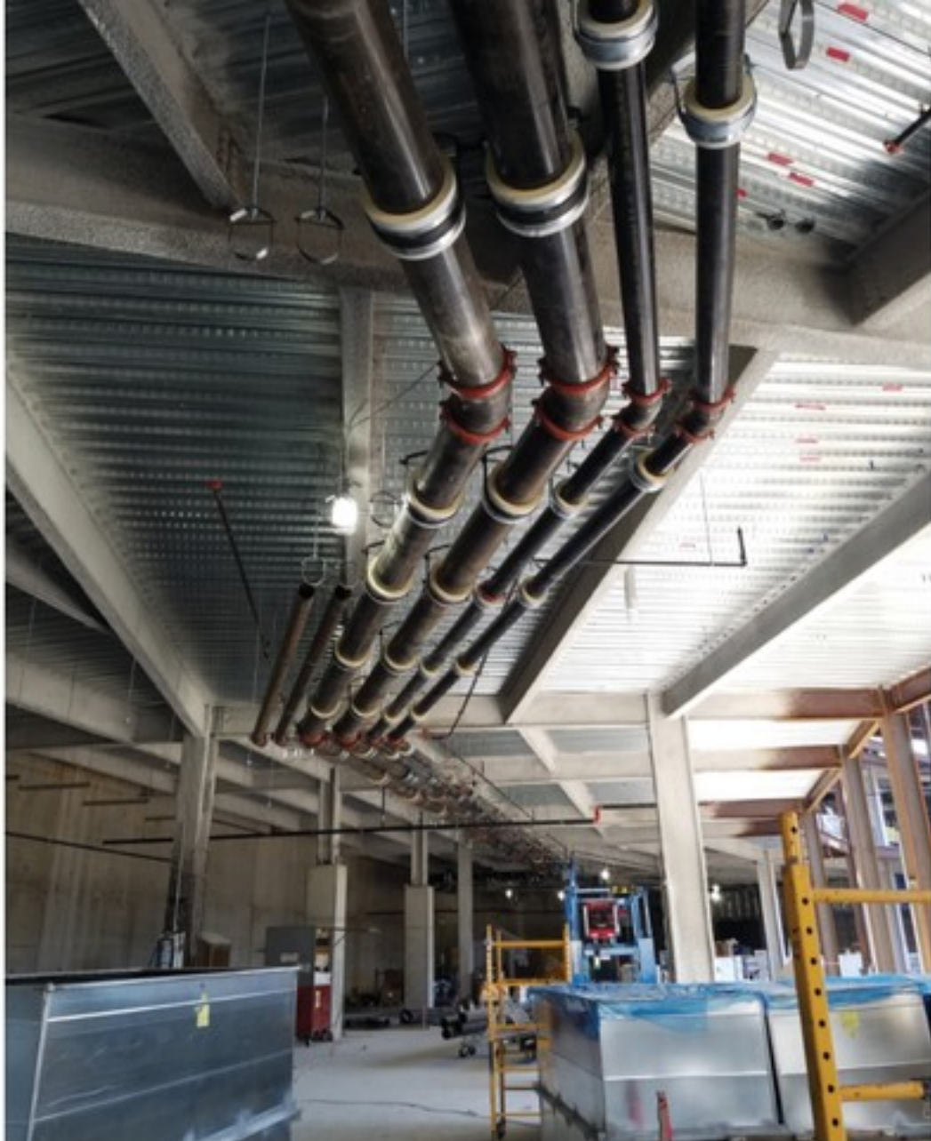
▲ The Event Level has 12-inch chilled water supply and return, six-inch heating hot water supply and return and food service heat recovery supply and return. Photo courtesy of Sellinger Associates
