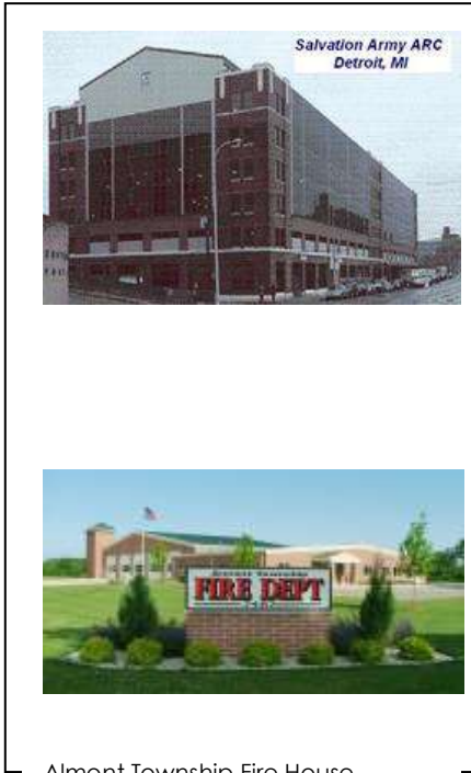
Almont Township Fire House
